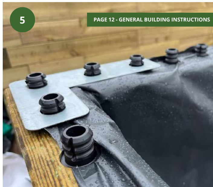
5 Install your angle corner plates - use your dowel protector to hammer these plates firmly into place.
