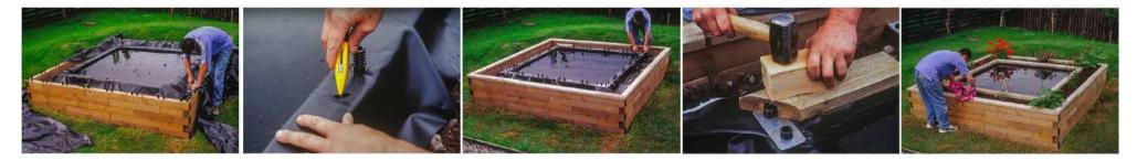
With a pond it's a good idea to pad the base of your build with carpet or sand to remove any sharp angles which could cause dirt build up. Next, ensure that the liner is fitted over the dowels, making a cross to allow the dowel through the pond liner. Finally, hook the liner to the top of the BlocX's prior to fitting the capping.
