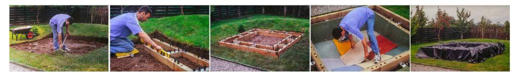
The key with any WoodBlocX build is to get the foundations level before you start. This allows you to easily build the layers of WoodBlocX as per your unique instruction pack (supplied with every kit).
